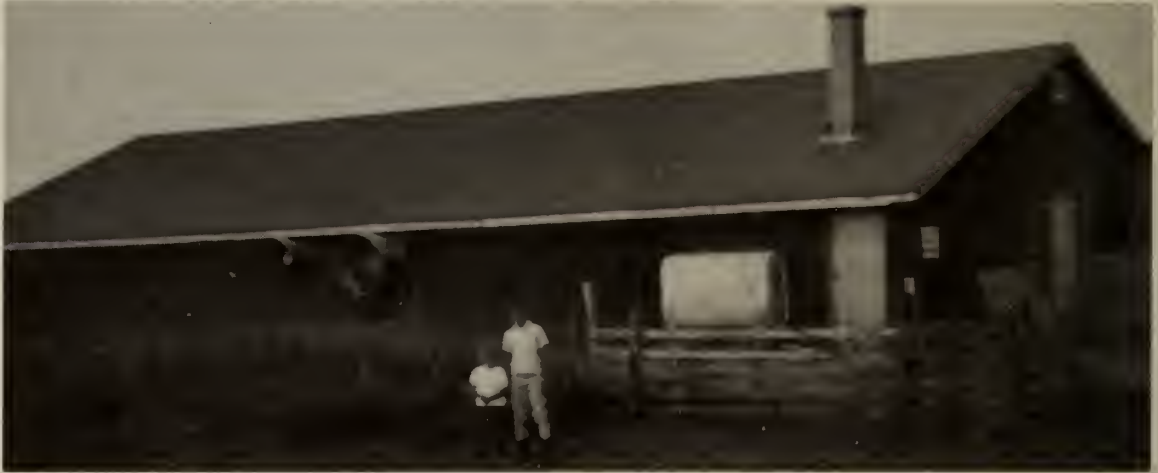
The first barn showing the Aerovent Ventilating System on the side.
